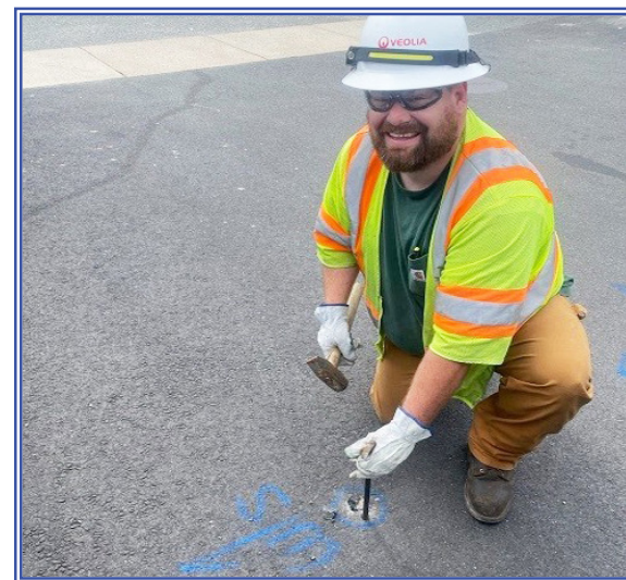
The exposure effort of a paved-over curb stop valve in Hyannis
